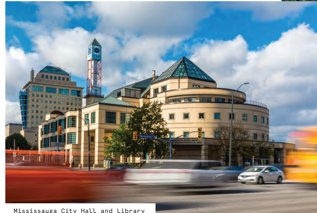
Mississauga City Hall and Library
